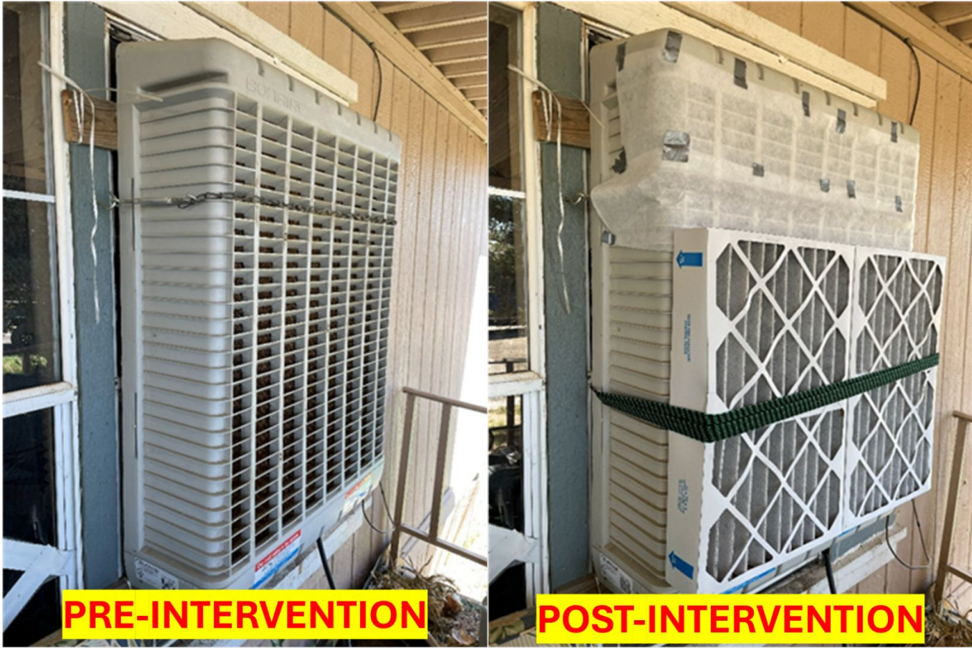
Figure A7. Combo DIY Solution – Regular Filters on EC combined with sheet filters due to EC shape irregularities and obstacles
