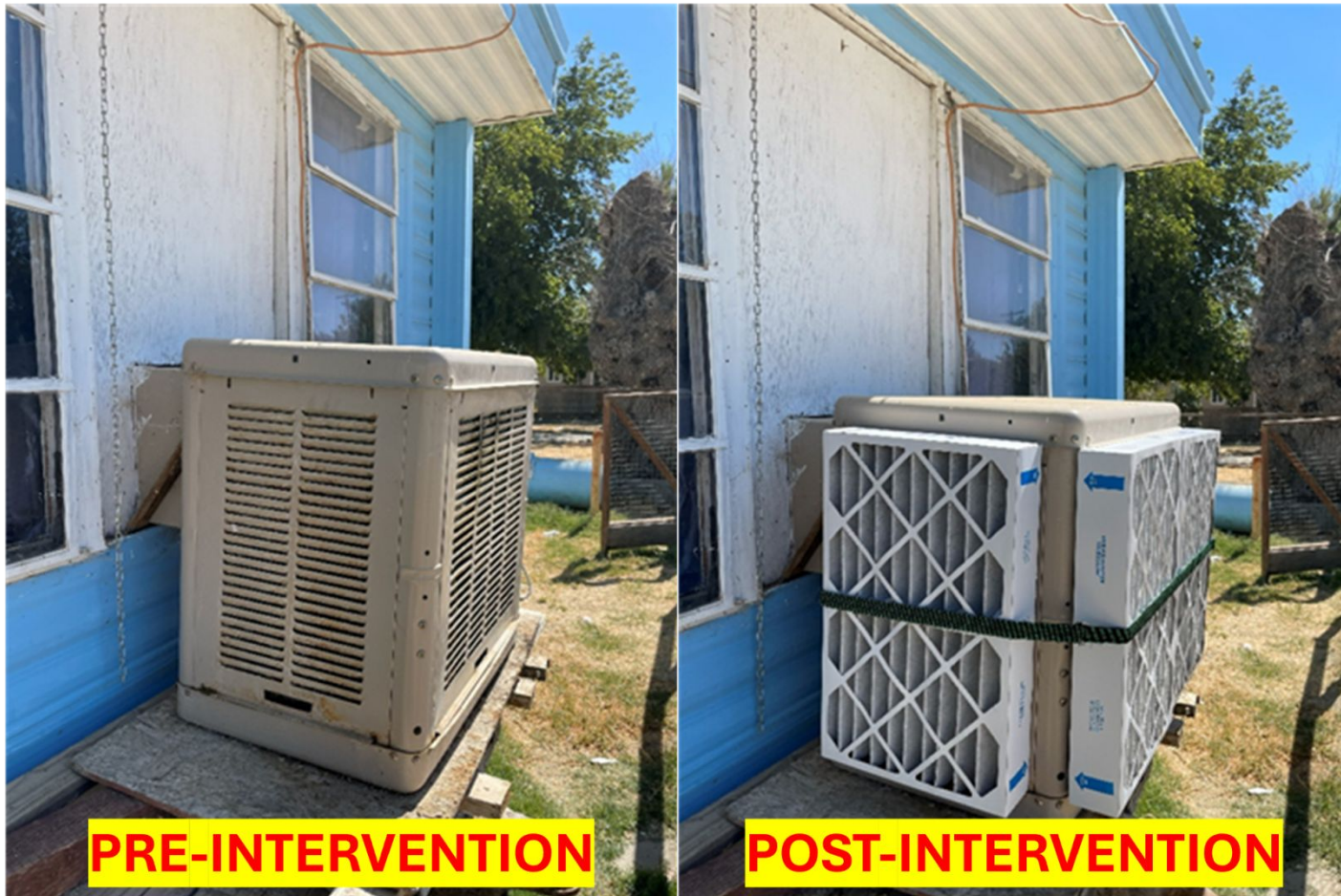
Figure A1. Regular DIY Solution – Filter dimensions conform closely to EC intakes with a bungee cord
