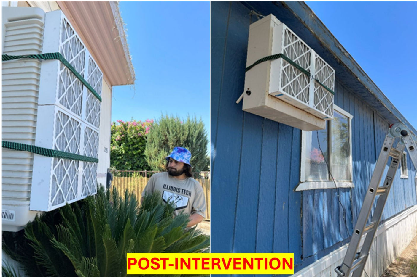
Figure A4. Regular DIY Solution - Filters on EC held together with a bungee cord but with some difficulties during installation due to surrounding obstacles
