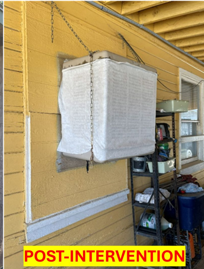
Figure A8. Sheet Filter Solution – Only Sheet filters on EC due to EC shape irregularities and obstacles preventing attachment of regular filters
