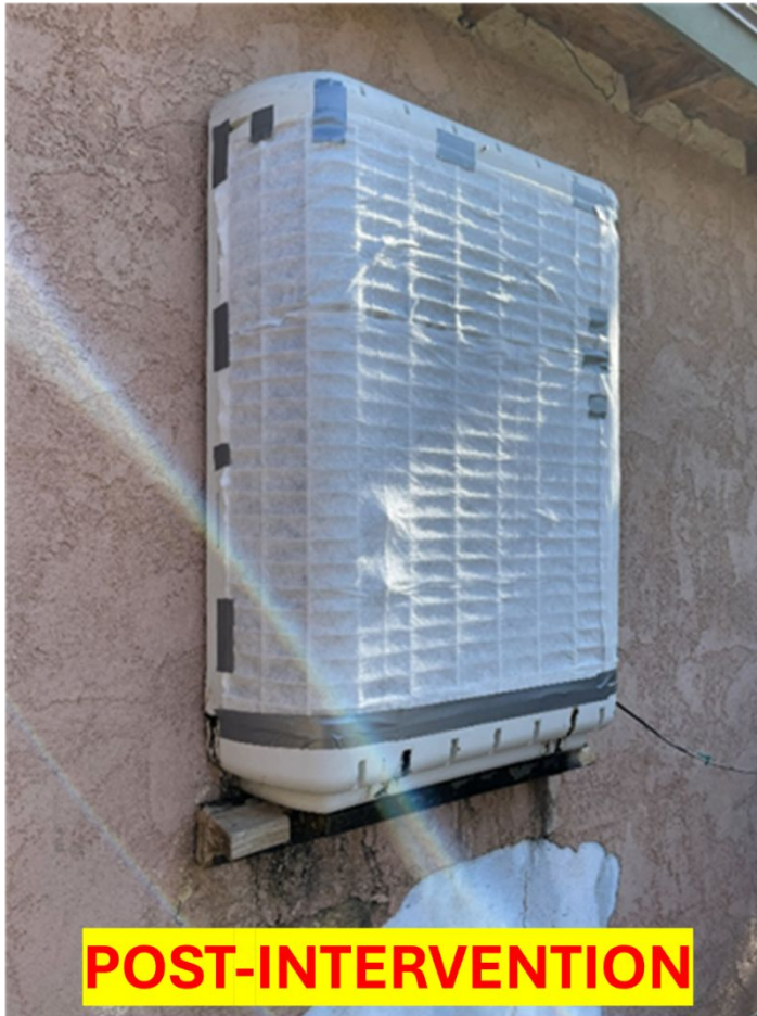
Figure A8. Sheet Filter Solution – Only Sheet filters on EC due to EC shape irregularities and obstacles preventing attachment of regular filters
