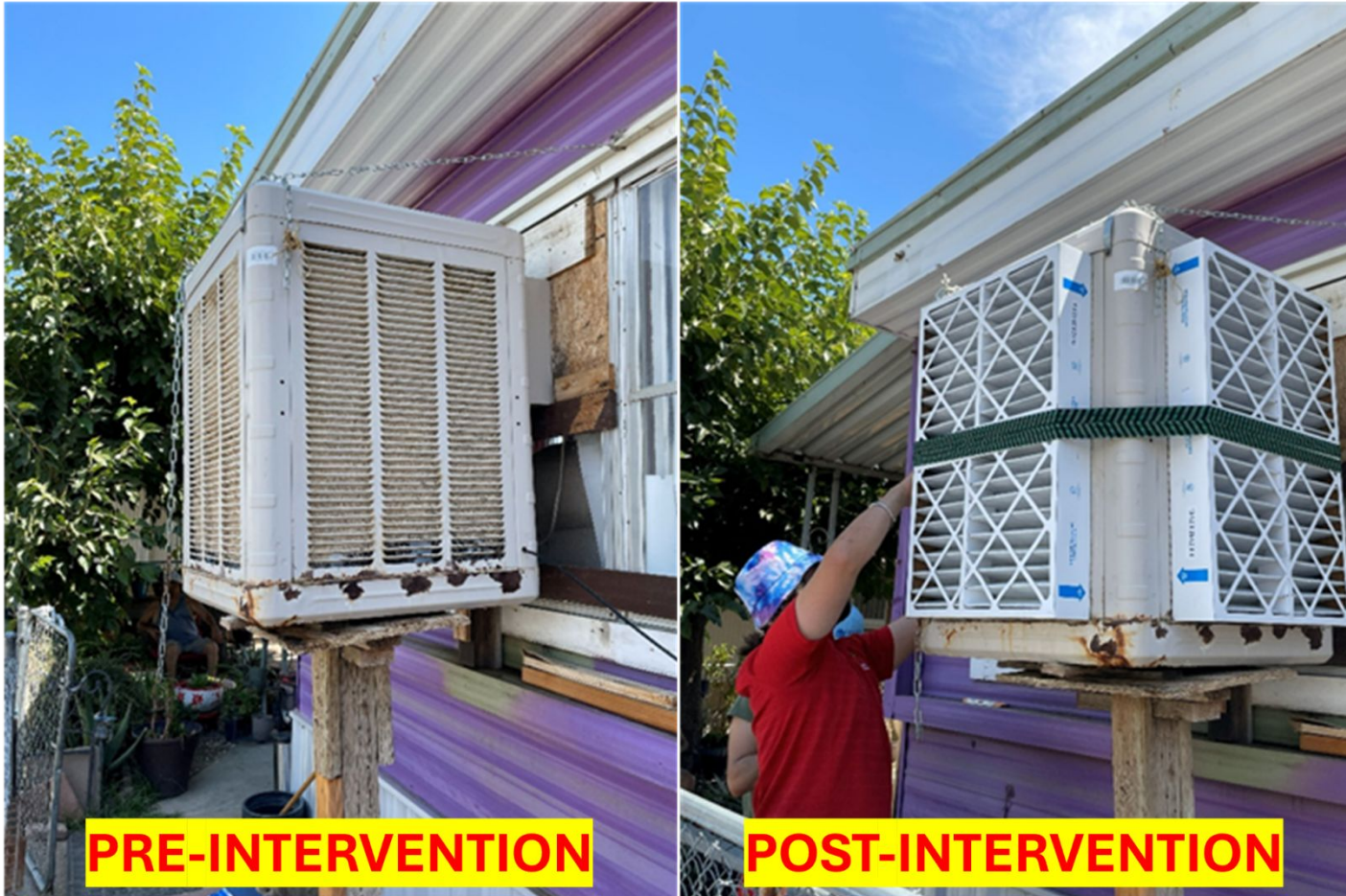
Figure A2. Regular DIY Solution - Filter dimensions conform closely to EC intakes with a bungee cord
