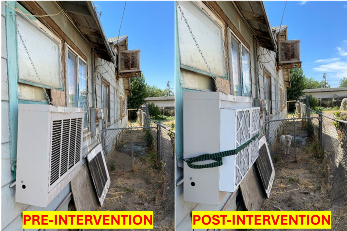
Figure A3. Regular DIY Solution - Filter dimensions conform closely to EC intakes with a bungee cord
