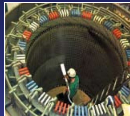
Stator Winding Cleaning
