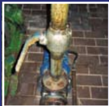
Dirt and grease build-up.
