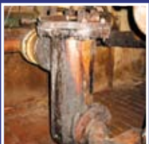
Dirt and grease build-up.
