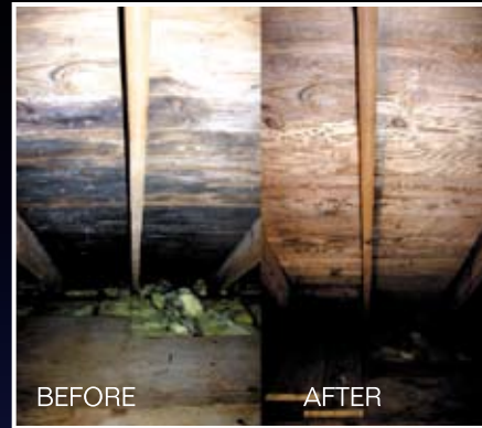
Cold Jet dry ice blasting removes 100% of mold spores from wood.
